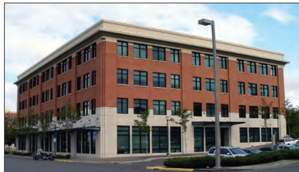
Barkley Office Buildings, Bellingham, WA
