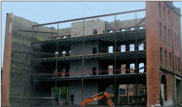
Historic Waldron Building Reconstruction
