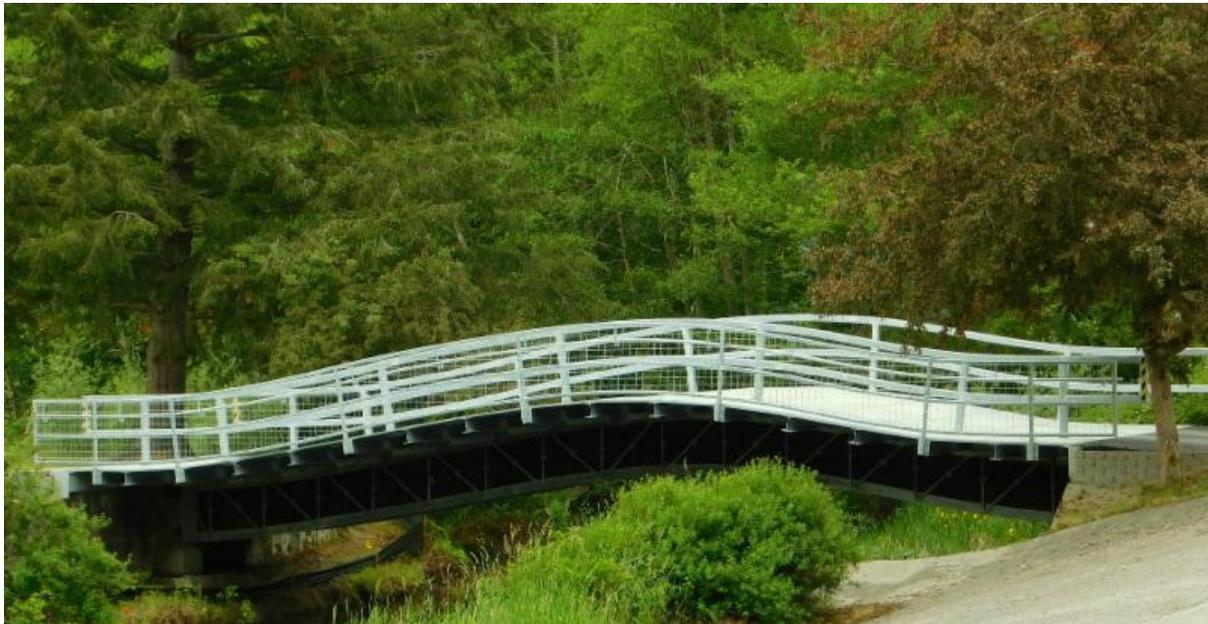
The completed bridge featuring steel support truss work, new deck and railings.
